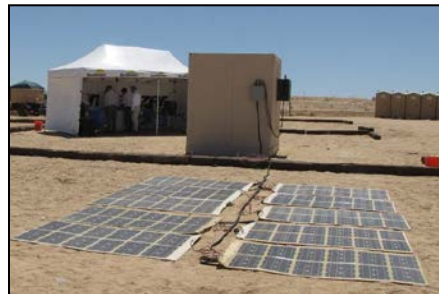
Solar cooling system
